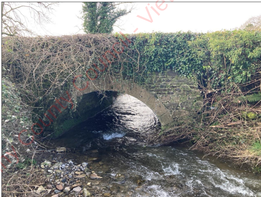
Plate 3-24. View of stone arched bridge crossing an EPA mapped watercourse classified as Eroding/upland river (FW1) along the Proposed Grid Connection underground cabling route.
