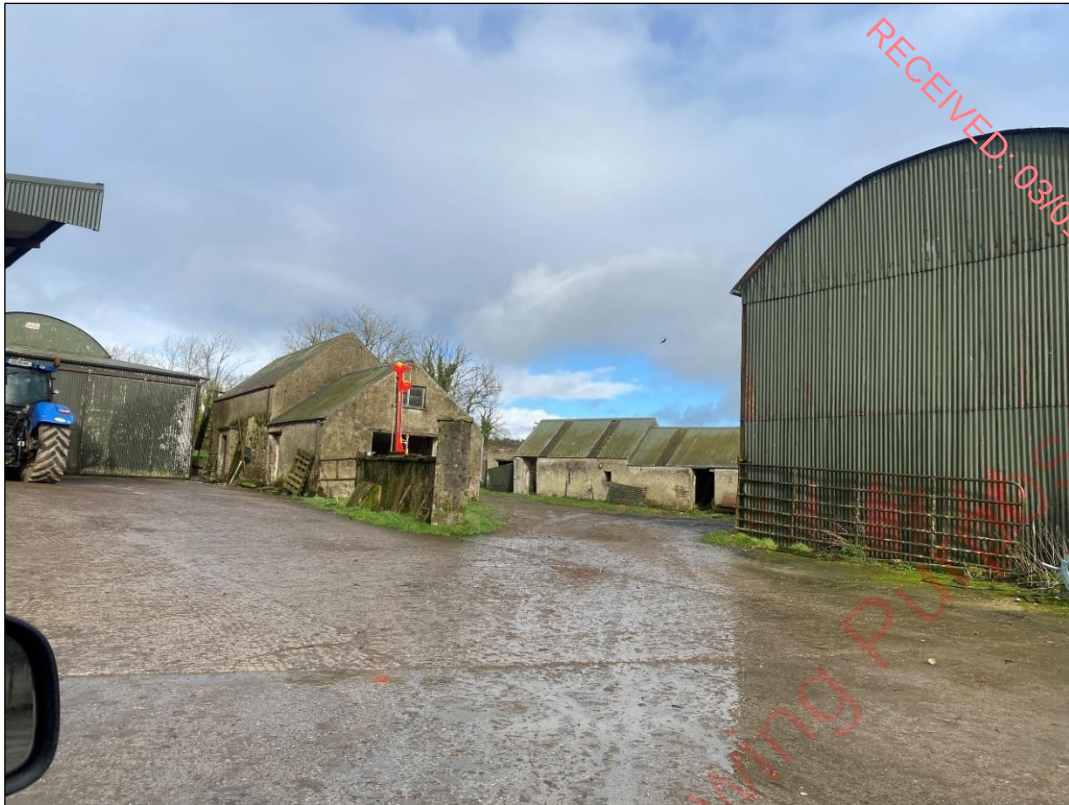
Plate 3-13. View of Buildings and artificial surfaces (BL3) located within the Proposed Wind Farm site.
