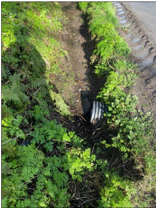
Plate 3-23. View of culvert beneath the road along the Proposed Grid Connection underground cabling route.
